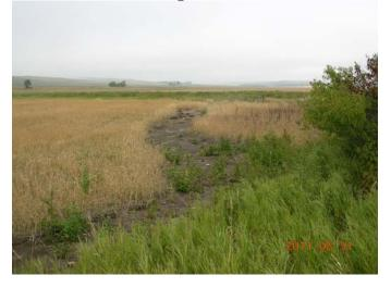
Original road ditch with Pond water overflow erosion visible on far end.
